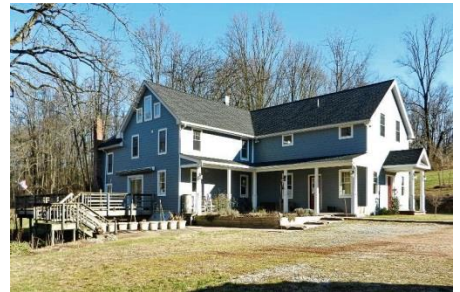
Renovations & Addition to 150-year old Farmhouse
