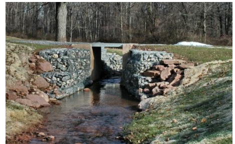
New Private Bridge with Gabion Wing Walls
